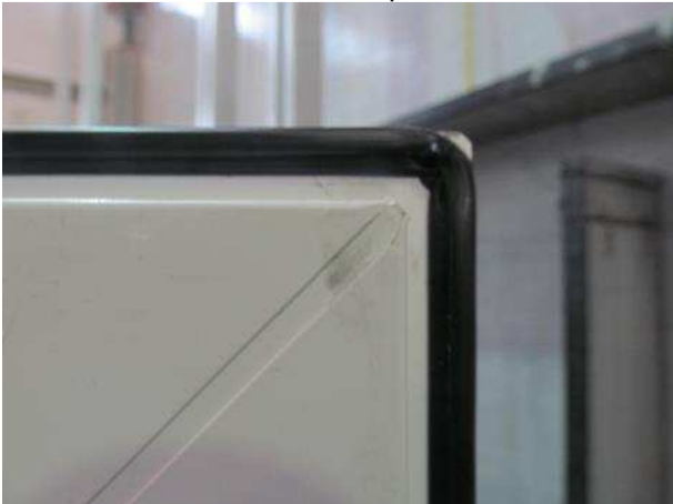
Picture 3 Rebate seal, external
