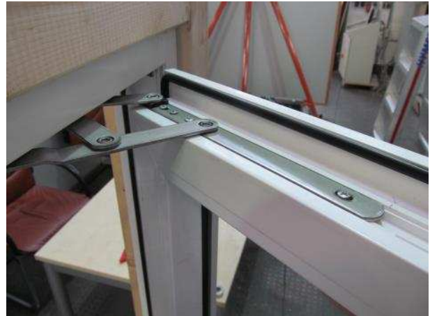
Picture 4 Tilt mechanism pivot, seen from rebate, frame
