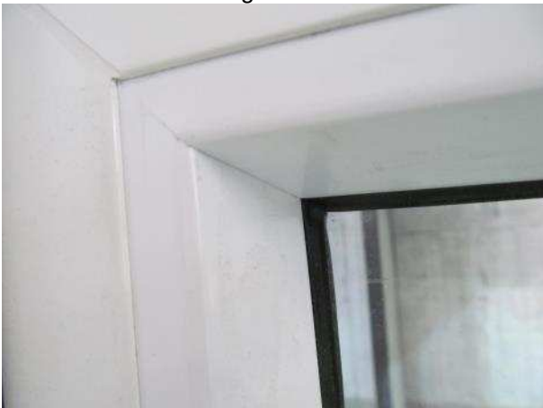
Picture 15 Fixing of the glazing internal
