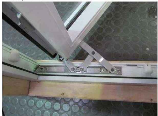
Picture 6 Corner pivot, seen from rebate
