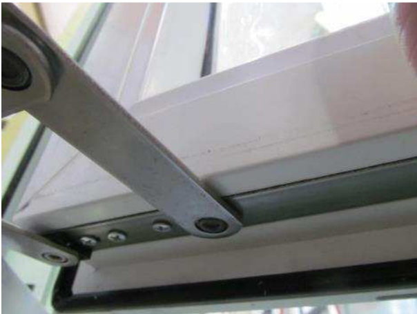
Picture 7 Corner pivot, seen from casement
