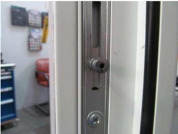
Picture 13 Locking situation casement 2
