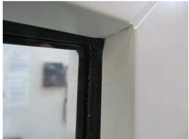
Picture 14 Fixing of the glazing external
