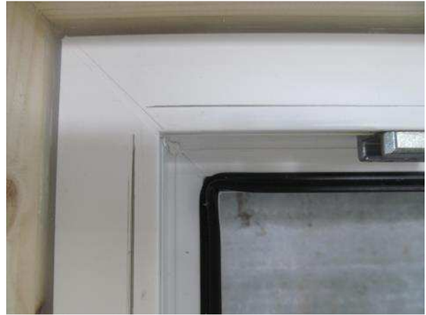
Picture 2 Rebate seal, internal
