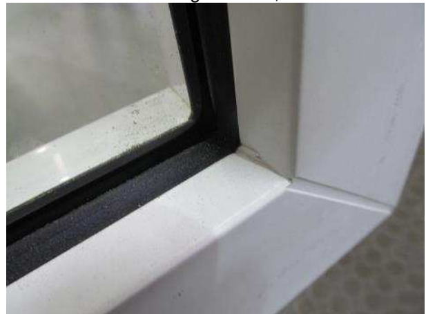
Picture 16 Fixing of the glazing external
