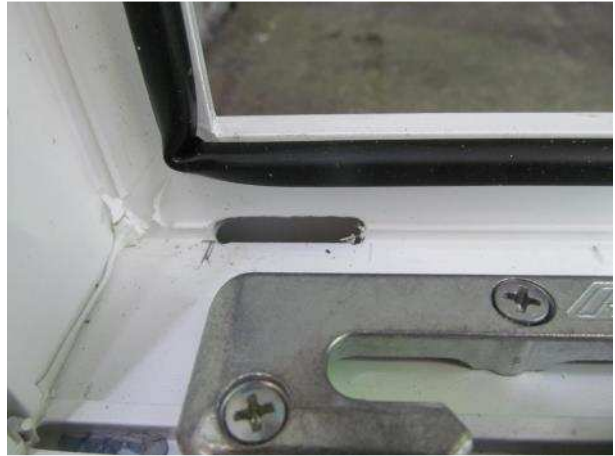
Picture 2 rebate seal, external
