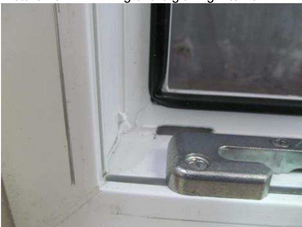
Picture 17 Drainage, seen from rebate
