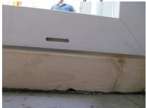
Picture 18 Drainage, seen from outside
