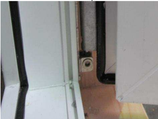
Picture 3 rebate seal, internal
