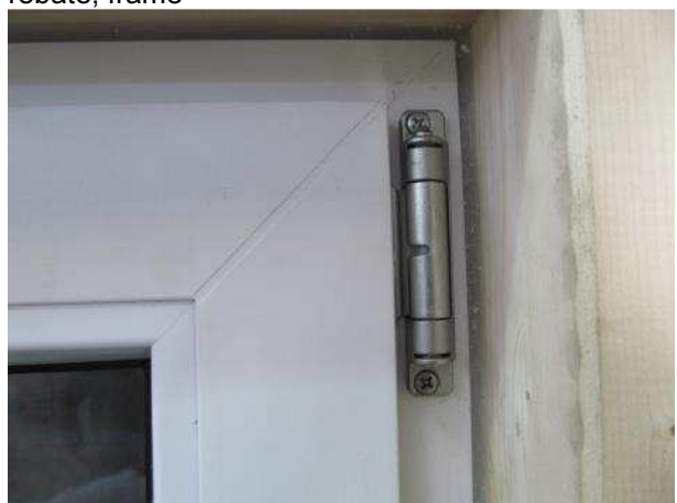
Picture 6 Tilt mechanism pivot, seen from inside
