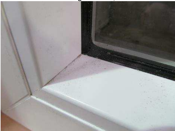
Picture 15 Fixing of the glazing internal
